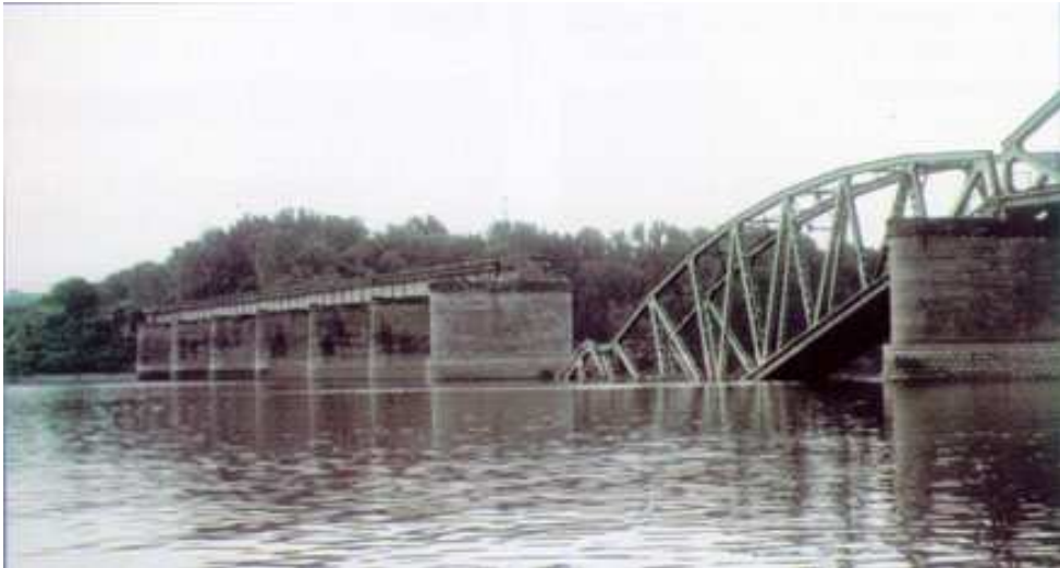
Figure 2.3 Destroyed railway bridge on the Sava.
